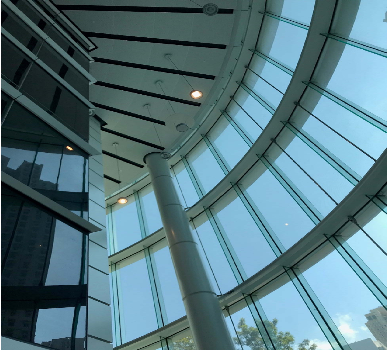
Figure 5.1.2 Redundant Luminaires Spotted in ACB
